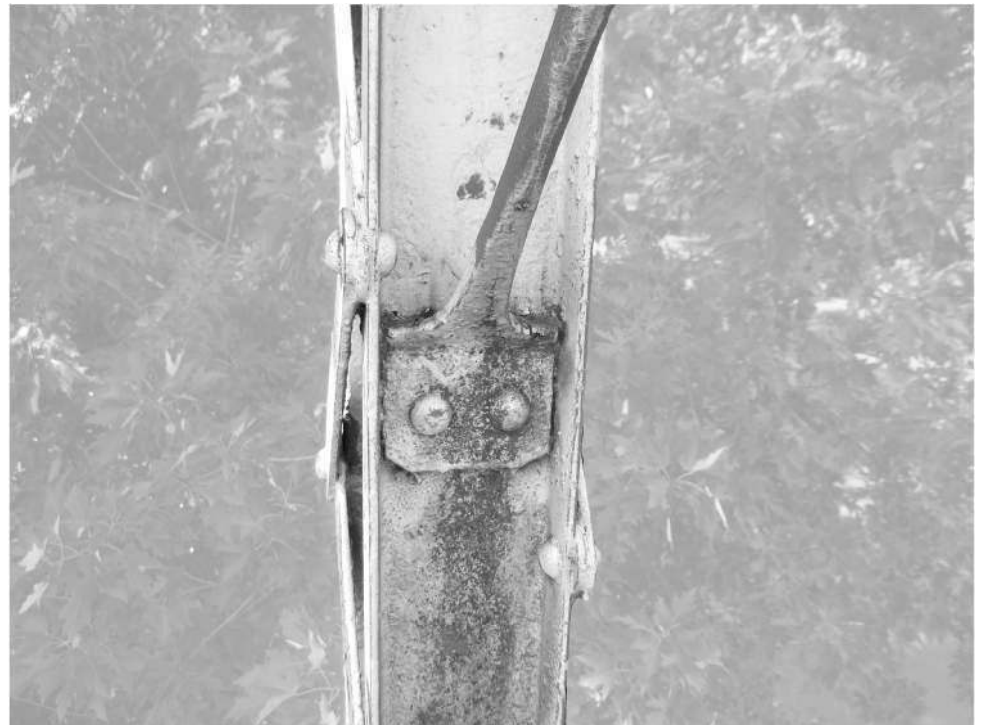
TYPICAL KNEE BRACE TO VERTICAL CONNECTION - SAVE AND REFURBISH CONNECTIONS. ** REPLACE RIVETS WITH HIGH STRENGTH BOLTS.
