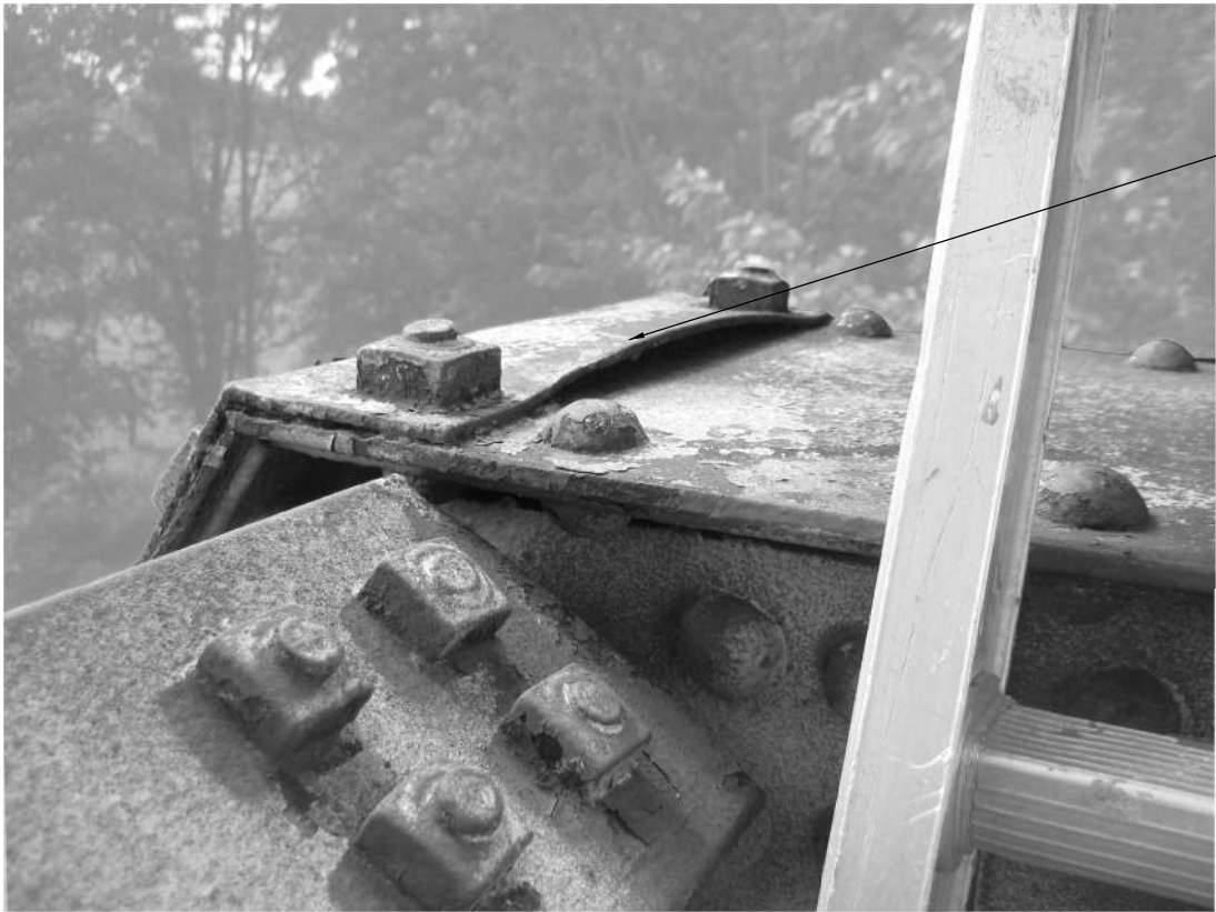
TYPICAL COVER PLATE AT END POST TO TOP CHORD CONNECTION ALL COVER PLATES SHALL BE REPLACED.
