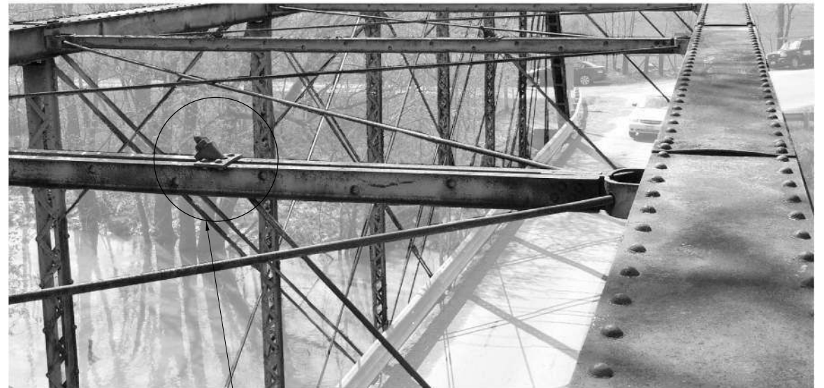
TYPICAL KNEE BRACE TO TOP STRUT CONNECTION ** CLEAN & GALVANIZE TOP STRUTS, LATERAL BRACES, KNEE BRACES INCLUDING CONNECTIONS.
