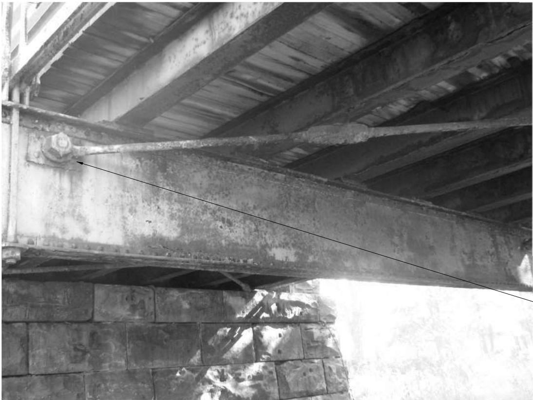
TYPICAL LOWER LATERAL BRACE TO FLOOR BEAM CONNECTION/ SAVE AND REFURBISH LOWER LATERAL BRACING/ (REPLACE BOLTS, NUTS, AND REINFORCEMENT PLATES AT LOWER LATERAL CONNECTION POINTS. USE EXISTING BOLT, NUT, AND WASHER SIZES AS PROTOTYPE FOR NEW HARDWARE.) *
