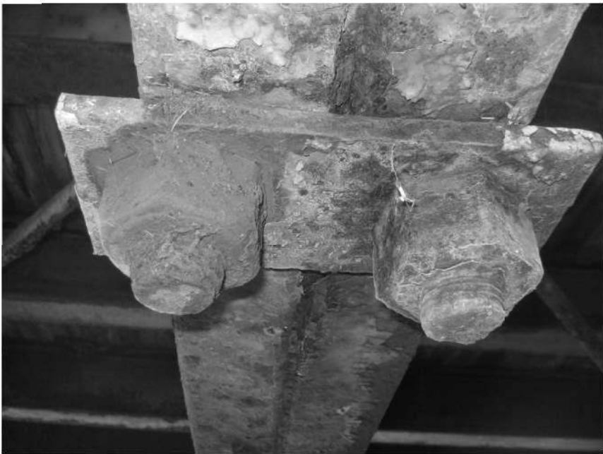
TYPICAL FLOOR BEAM TO TRUSS HANGER BOLT & PLATE REPLACE ALL HANGER BOLTS, NUTS, AND PLATES. SEE SHEET 40/52 FOR HANGER BOLT & PLATE DETAILS.
